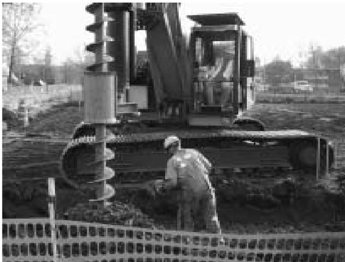
*An auger is used to dig pilot holes and loosen the soil before beginning piledriving.*
