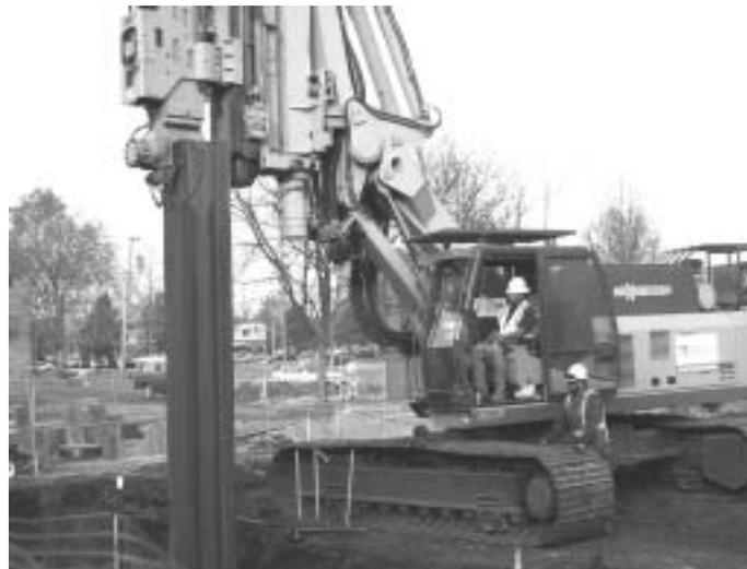
*Interlocking 50-ft steel pilings are vibration-driven into the soil prior to excavation.*
